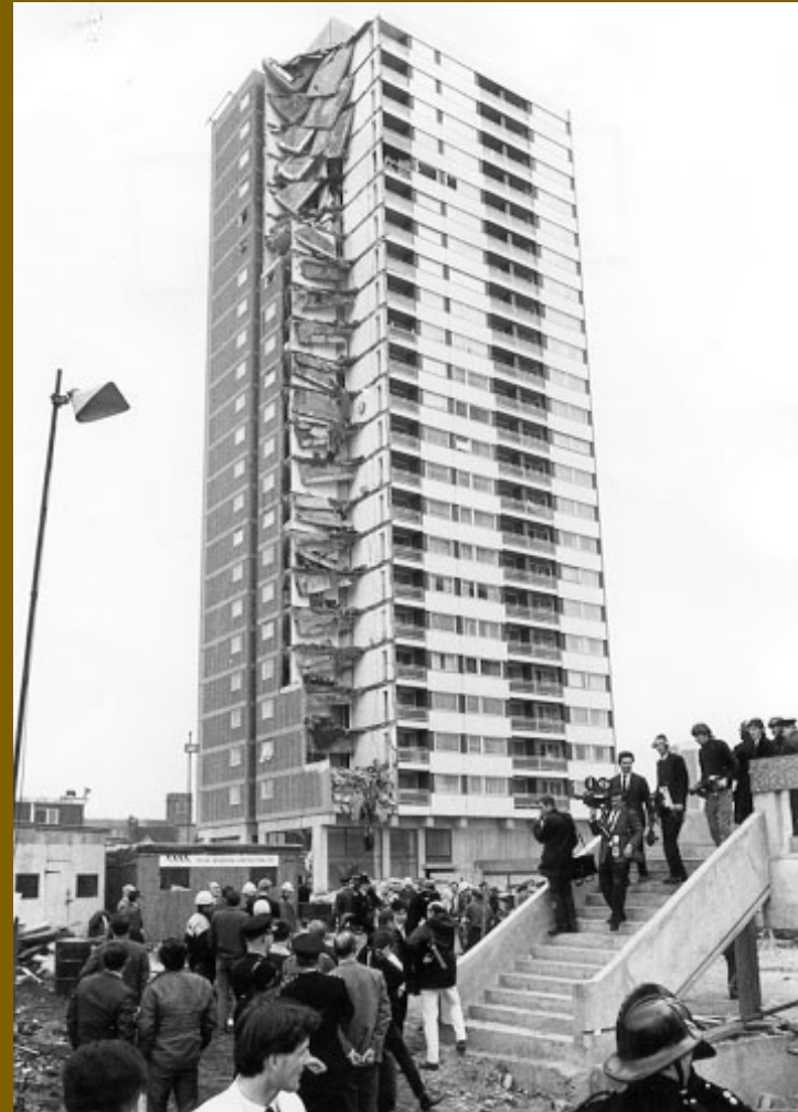
Ronan Point, following the gas explosion.
