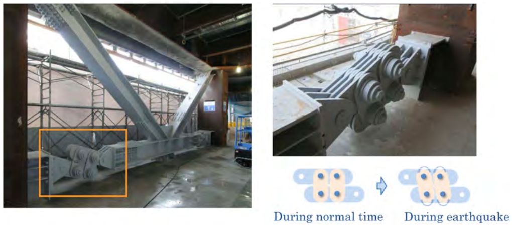
Figure 28. Appearance of rotational friction damper.
