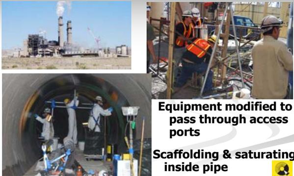
Equipment modified to pass through access ports
