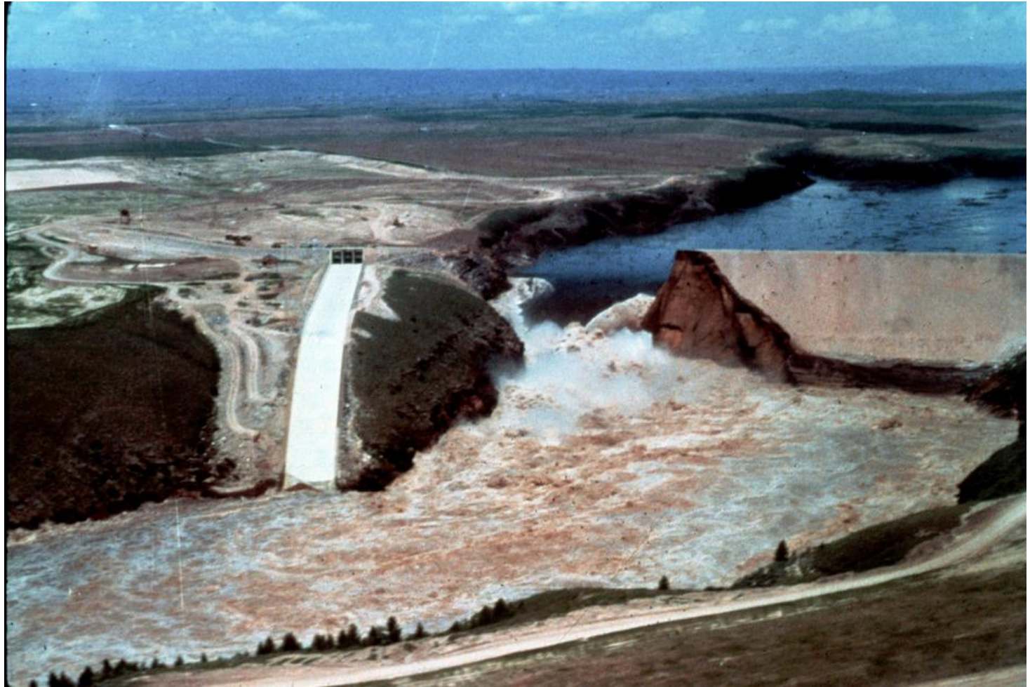
Teton Dam Failure, 1976
