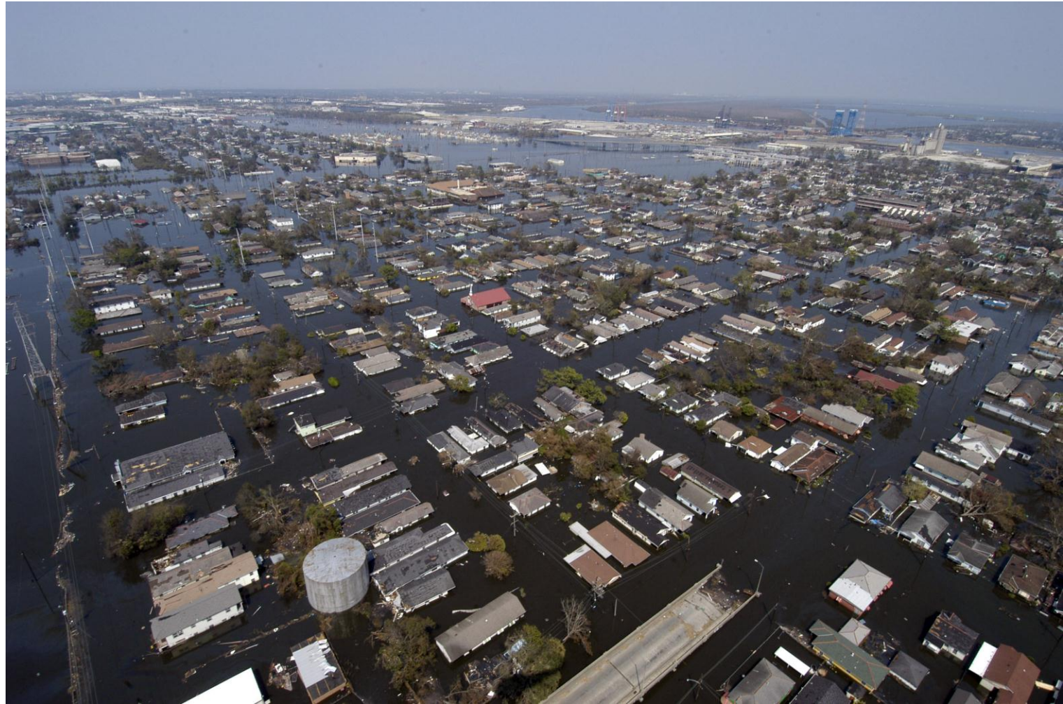
Hurricane Katrina, New Orleans, 2005
