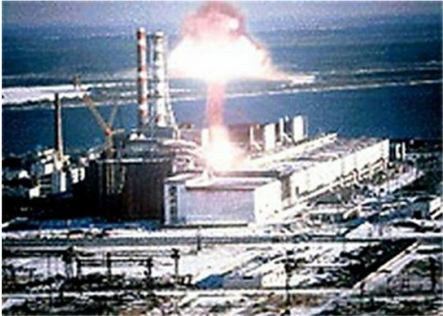
Chernobyl Nuclear Power Plant, 1986
