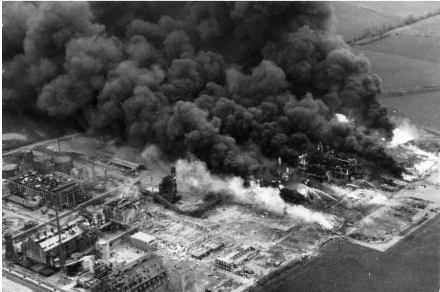
Flixborough Chemical Plant, 1974
