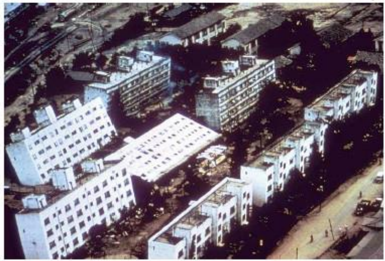
Figure 1: Soil liquefaction during earthquake shaking – (a) Process of liquefaction, and (b) Collapse of buildings during 1964 Niigata Earthquake
