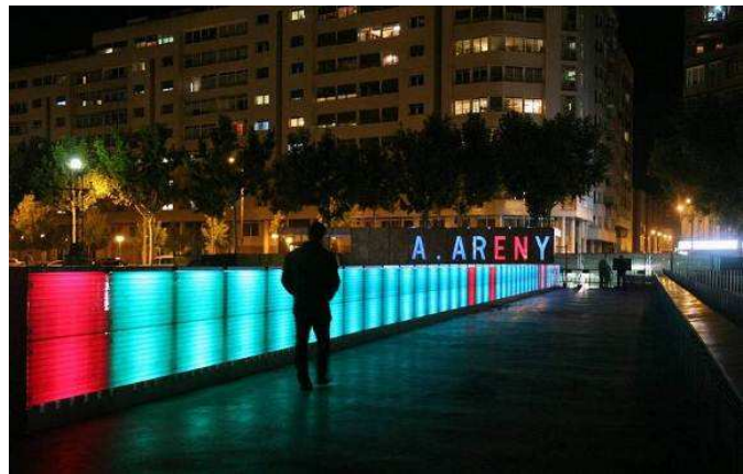
Fig. 11. Railings with GFRP panels.
