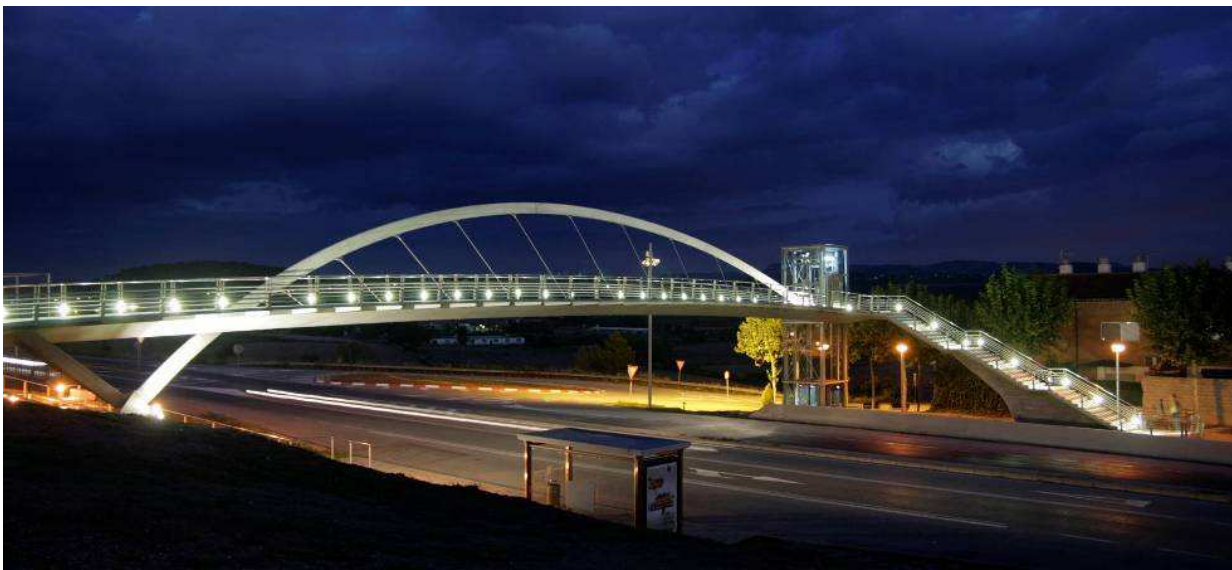
Fig. 1 Sant Fruitós Footbridge.
