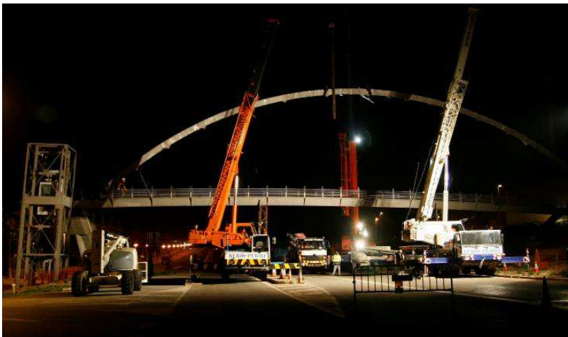
Fig. 3 Sant Fruitos Footbridge. Assembly of the arch.
