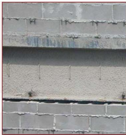
Figure 15: Locate bond beam directly under steel beam only if there is room to grout from the exterior side
