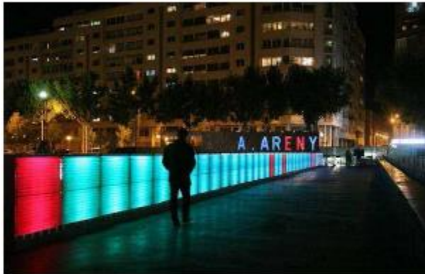
Fig. 11. Railings with GFRP panels.
