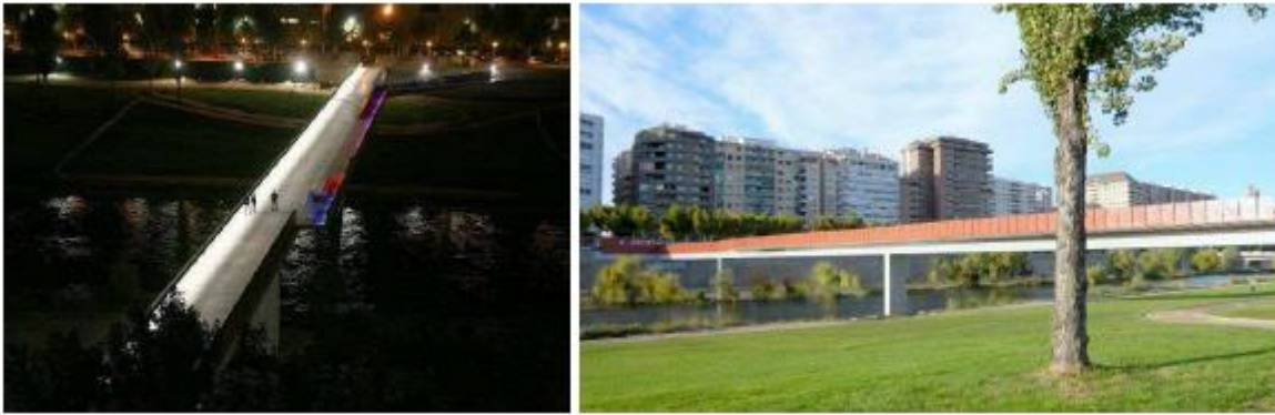
Figs. 8 and 9 Footbridge over Segre River. General views.
