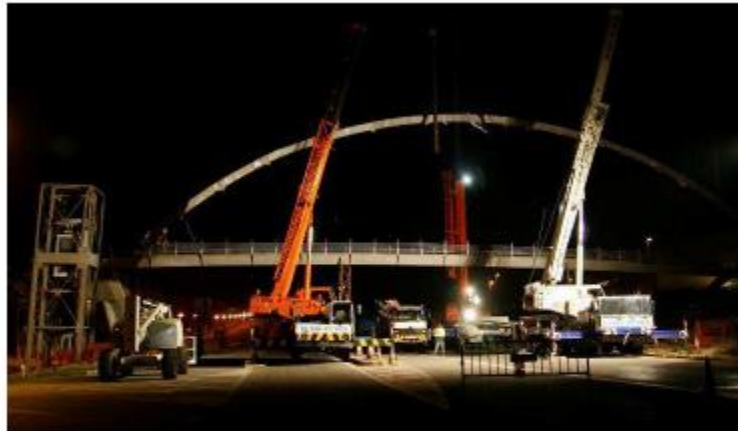
Fig. 3 Sant Fruitos Footbridge. Assembly of the arch.
